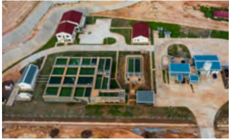
Municipal wastewater treatment plant in Kumasi, Ghana Capacity: 1,000 m 3 /d Budget: 10€ million
